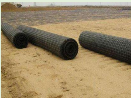
Exposed Biaxial Plastic Geogrid
