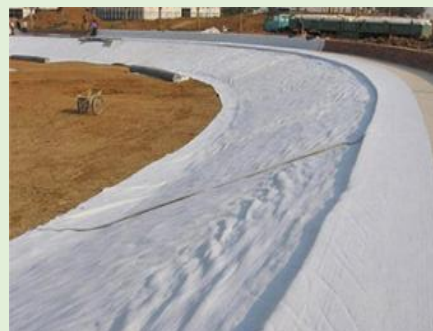
Spot-storing Geotextile
