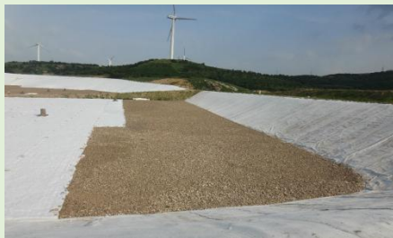
Exposed geotextile
