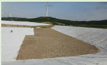
Exposed geotextile
