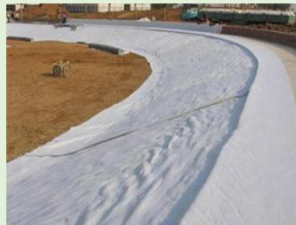
Spot-storing Geotextile
